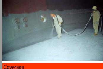
UPC-6001 is applied in continuous coats from 10 to 250 mils, and has no limit on thickness buildup.
