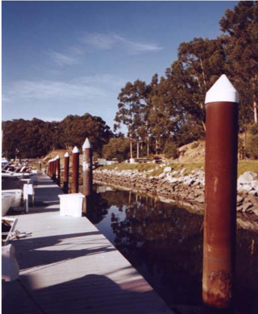
UNCOATED STEEL PILE
